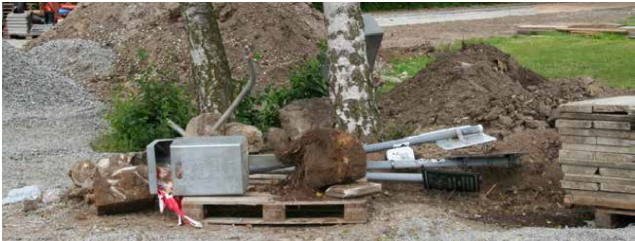
Figure 4.12: Damage to the trunk and root area that can be avoided by tree protection (Thieme-Hack)
